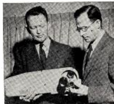
NEW CBS color camera chain, which is one-sixth the size and one-third the weight of present black-and-white cameras, is held by James Reeves (l), CBS engineer, as Dr. Peter Goldmark, the network's director of engineering and research development, inspects the unit.
